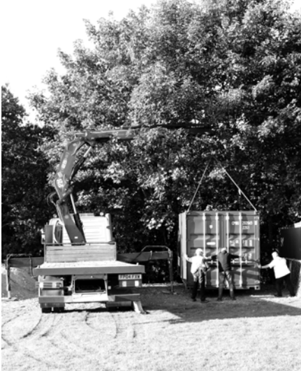
A slight addition to the landscape at the Sports Field as a new equipment storage facility is lowered into place. See Page 5.
